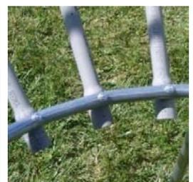
*Attaching columns to upper and lower rings*
